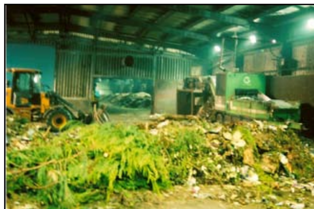
Green waste reception area with compost heaps in the background
